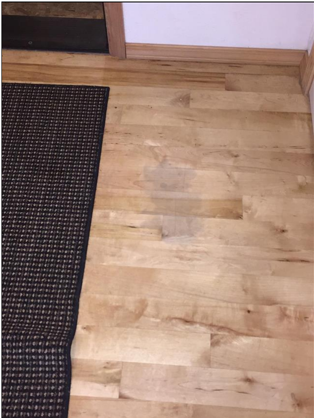
5.2 Item 2(Picture) Moisture staining
