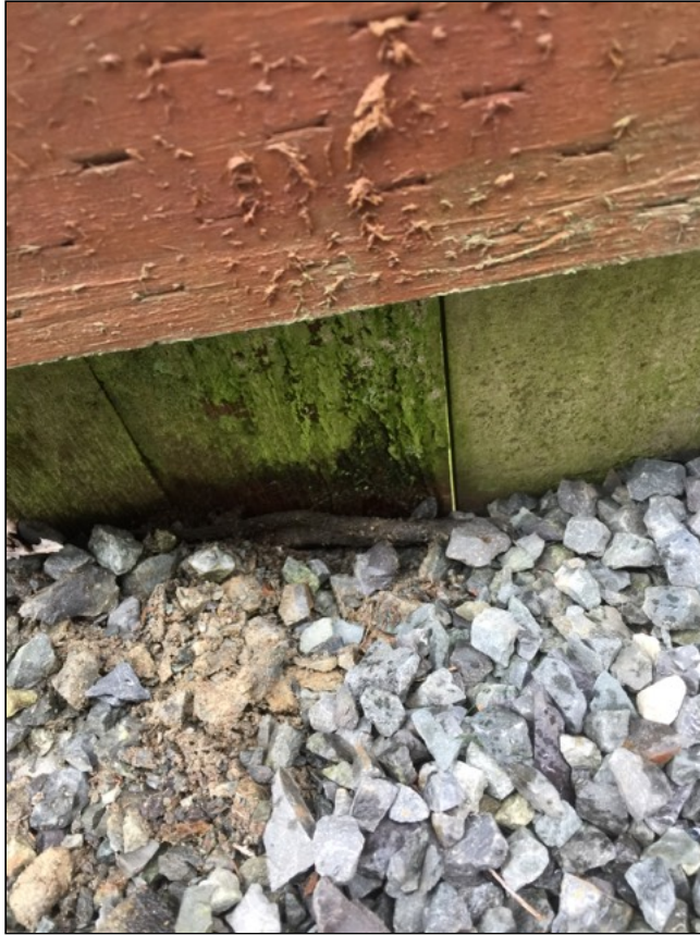
1.3 Item 1(Picture) Fence board wood decay
