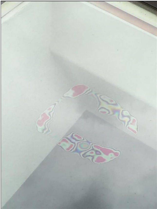
2.2 Item 2(Picture) Skylight defect
