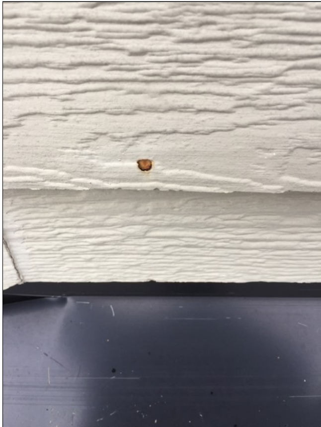
1.0 Item 6(Picture) Exposed nail heads
