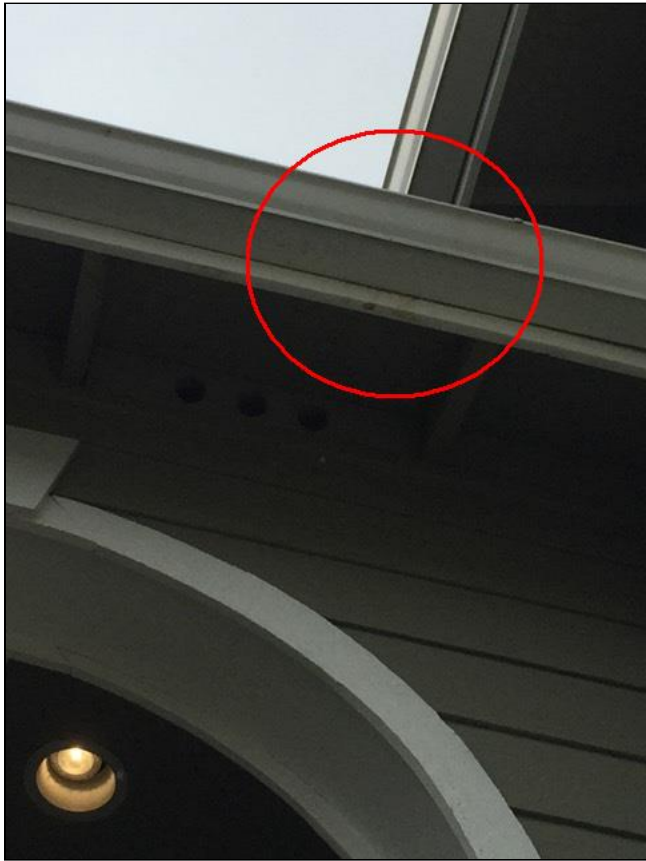
1.5 Item 1(Picture) Possible moisture behind gutter.
