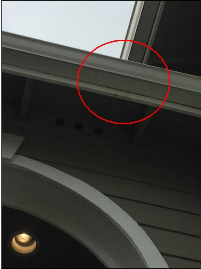
1.5 Item 1(Picture) Possible moisture behind gutter.
