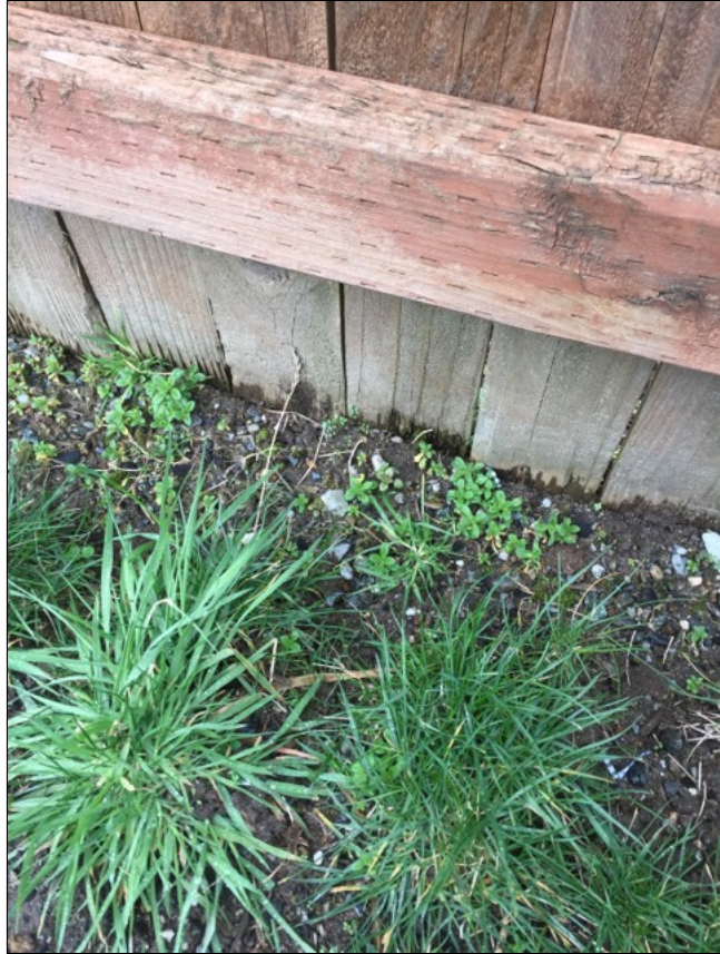
1.3 Item 2(Picture) Wood to soil contact
