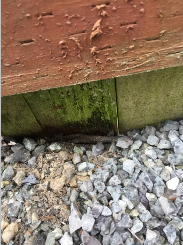
1.3 Item 1(Picture) Fence board wood decay
