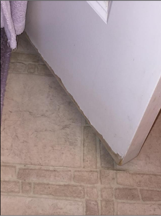
4.3 Item 3(Picture) Bottom of bathroom door damage
