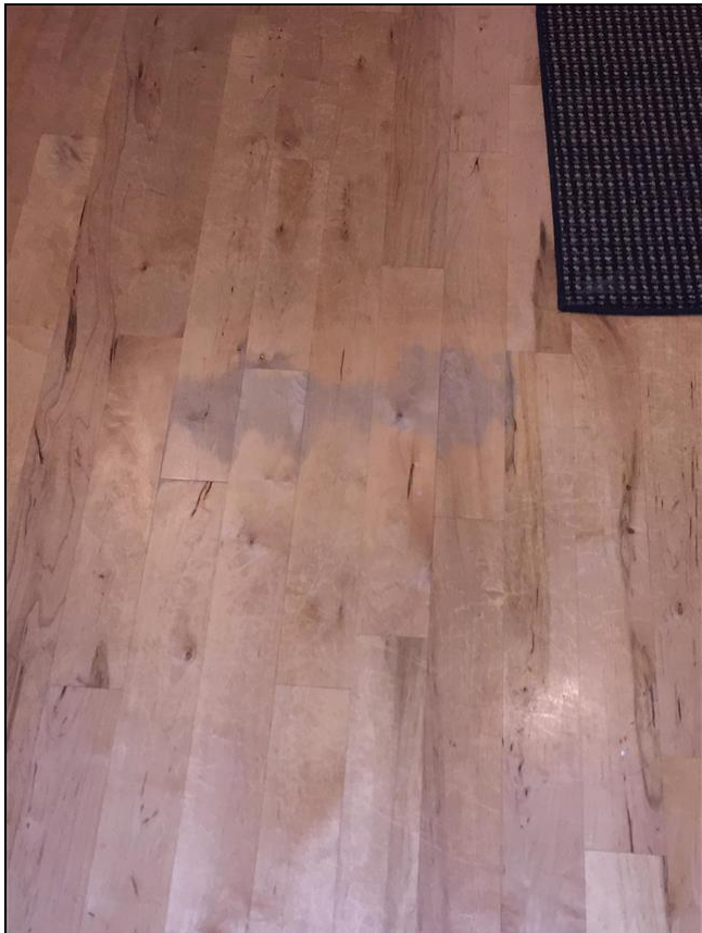
5.2 Item 1(Picture) Moisture staining
