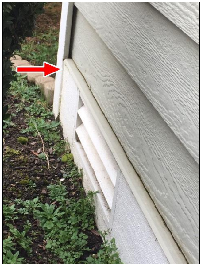
1.0 Item 2(Picture) Flashing at the SE corner
