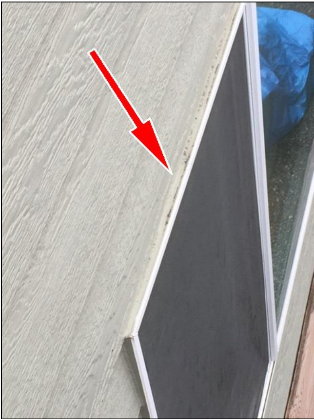
1.0 Item 7(Picture) No flashing
