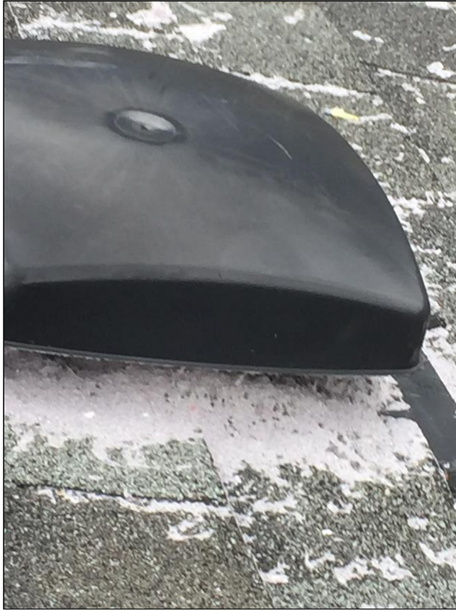
2.3 Item 1(Picture) Dryer venting lint onto the roof
