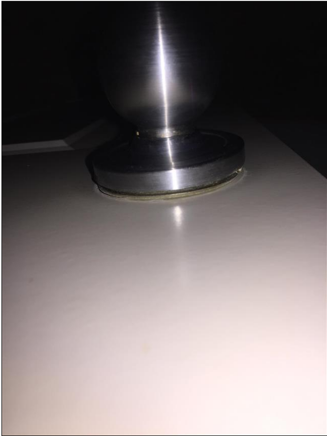
5.0 Item 2(Picture) Loose door knob plate
