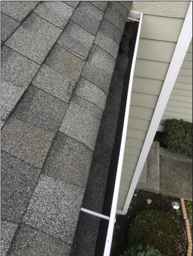
2.0 Item 2(Picture) Gutters full of granules
