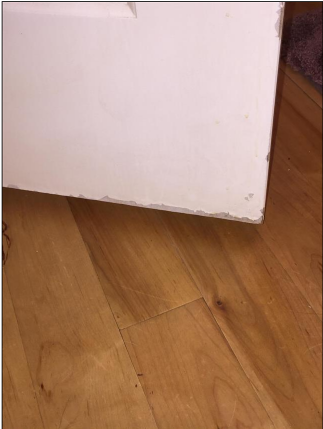
4.3 Item 1(Picture) Bottom of bathroom door damage
