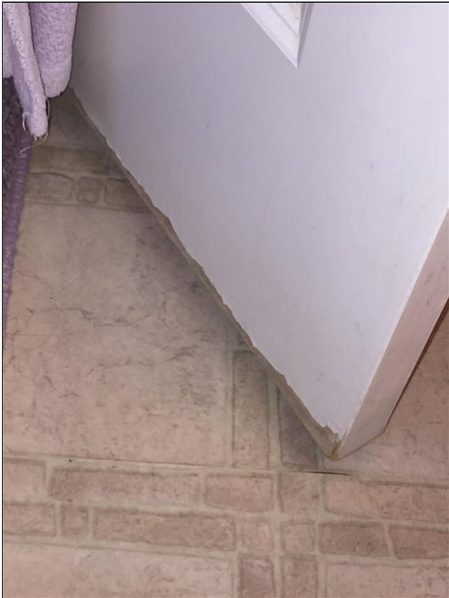
4.0 Item 2(Picture) Bathroom door moisture damage
