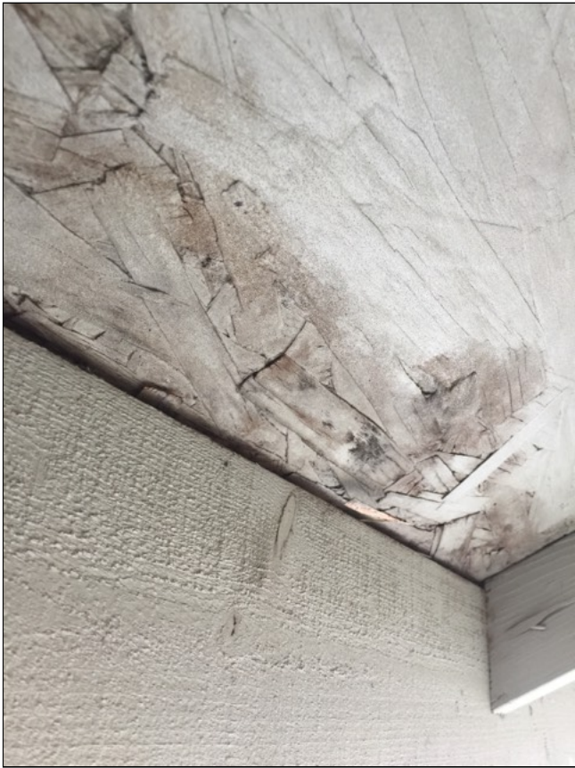
1.5 Item 2(Picture) Moisture staining behind gutter and fascia
