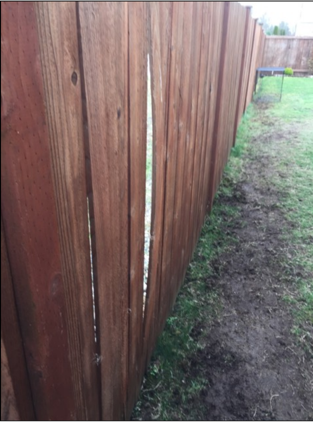
1.3 Item 3(Picture) Warped fence boards
