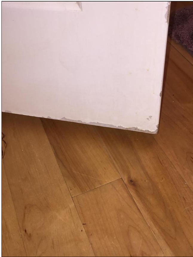
4.0 Item 4(Picture) Bathroom door moisture damage
