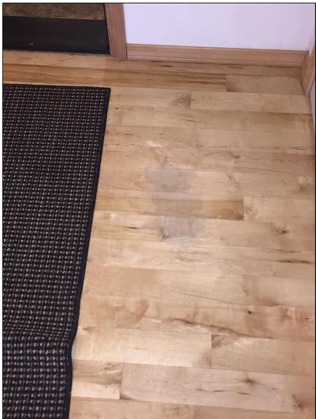
5.2 Item 2(Picture) Moisture staining
