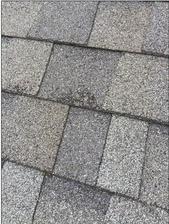
2.0 Item 1(Picture) Roof granuals missing
