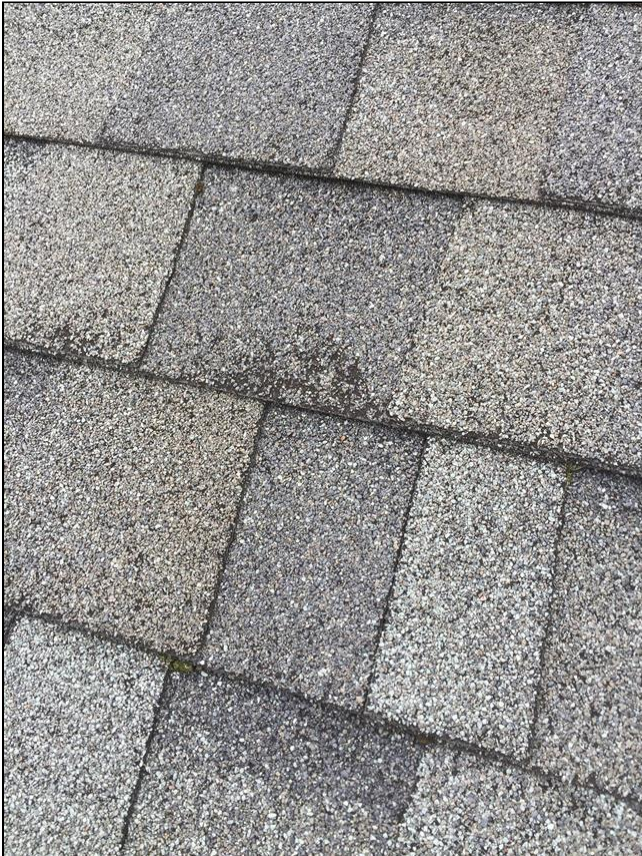
2.0 Item 1(Picture) Roof granuals missing
