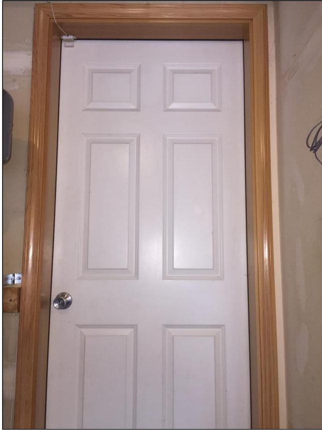
7.5 Item 1(Picture) Occupant door not self closing
