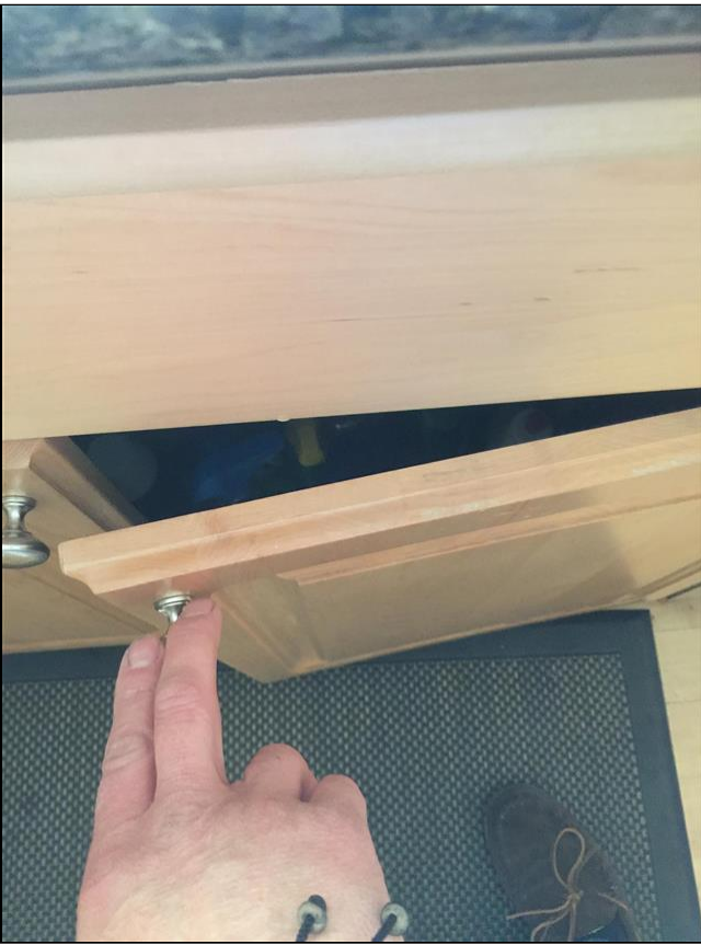
3.5 Item 1(Picture) Warped cabinet door under the sink
