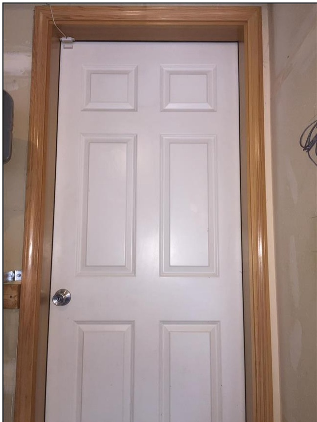
7.5 Item 1(Picture) Occupant door not self closing
