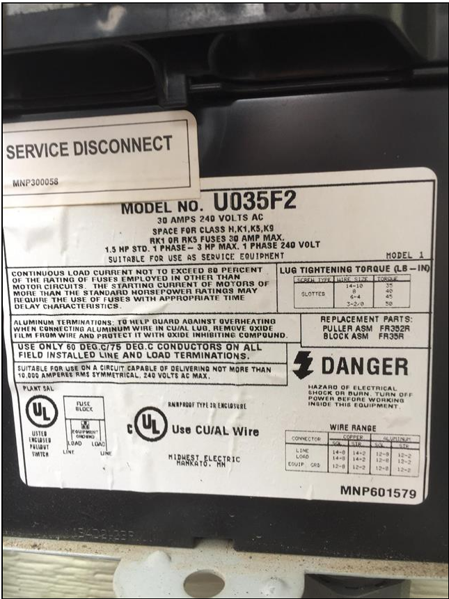
10.0 Item 3(Picture) service disconnect for air conditioner
