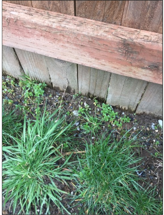
1.3 Item 2(Picture) Wood to soil contact
