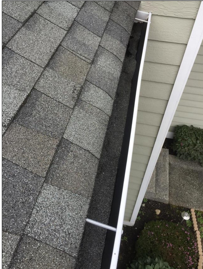
2.0 Item 2(Picture) Gutters full of granules
