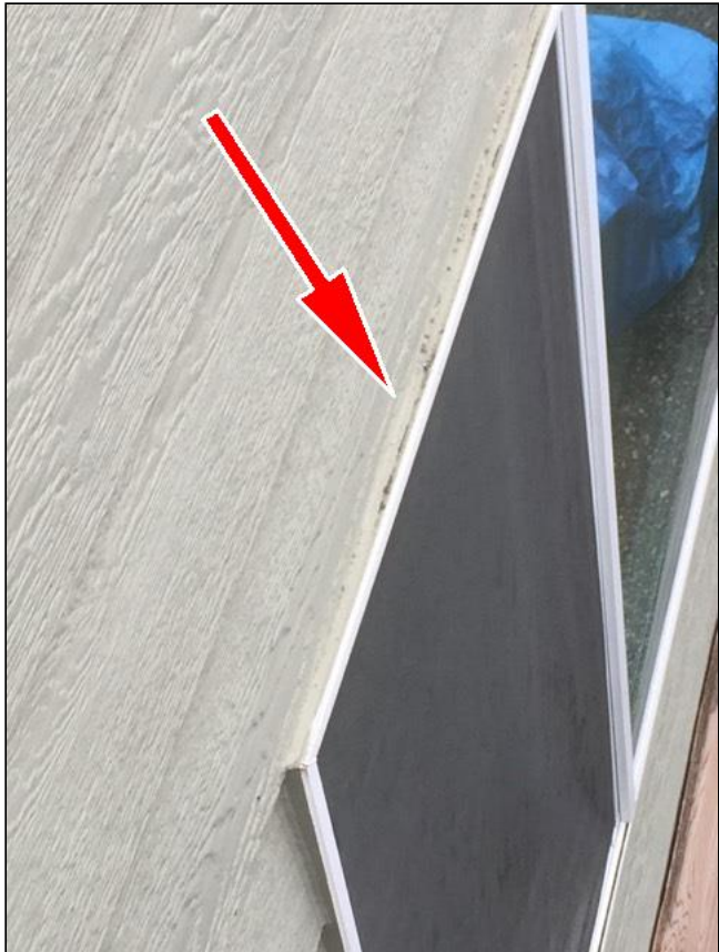
1.0 Item 7(Picture) No flashing
