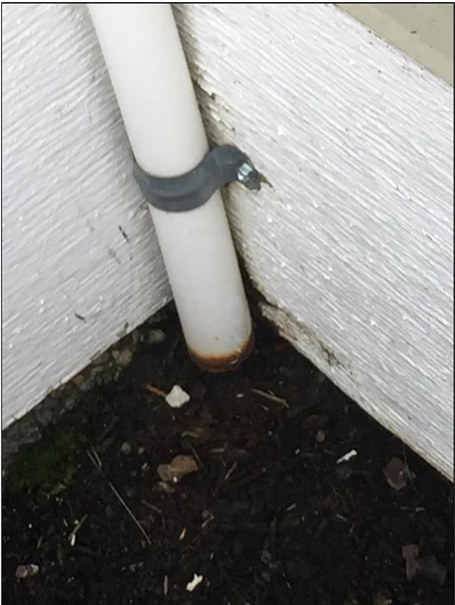
1.0 Item 10(Picture) Trim boards behind the TPR valve pipe
