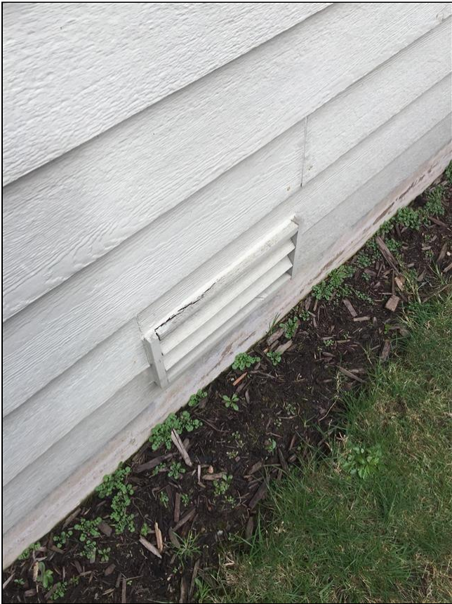
1.0 Item 9(Picture) Vent trim board damage
