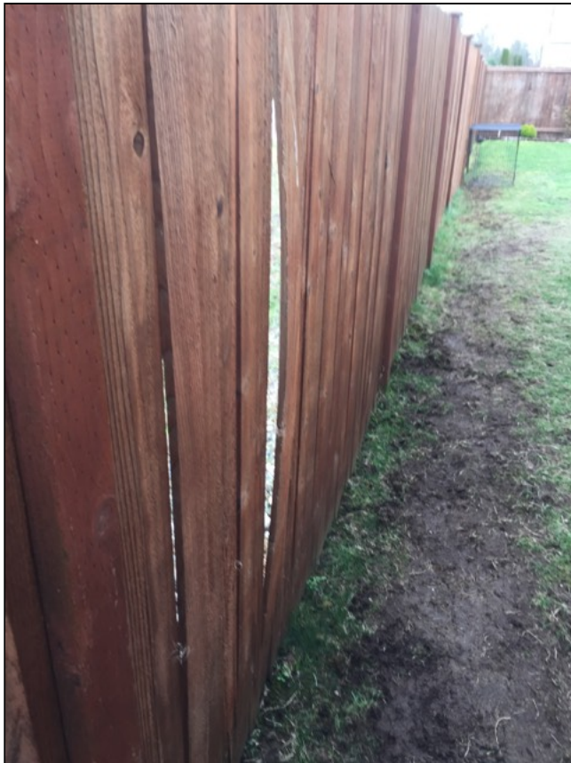
1.3 Item 3(Picture) Warped fence boards
