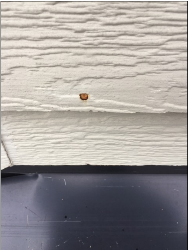
1.0 Item 6(Picture) Exposed nail heads
