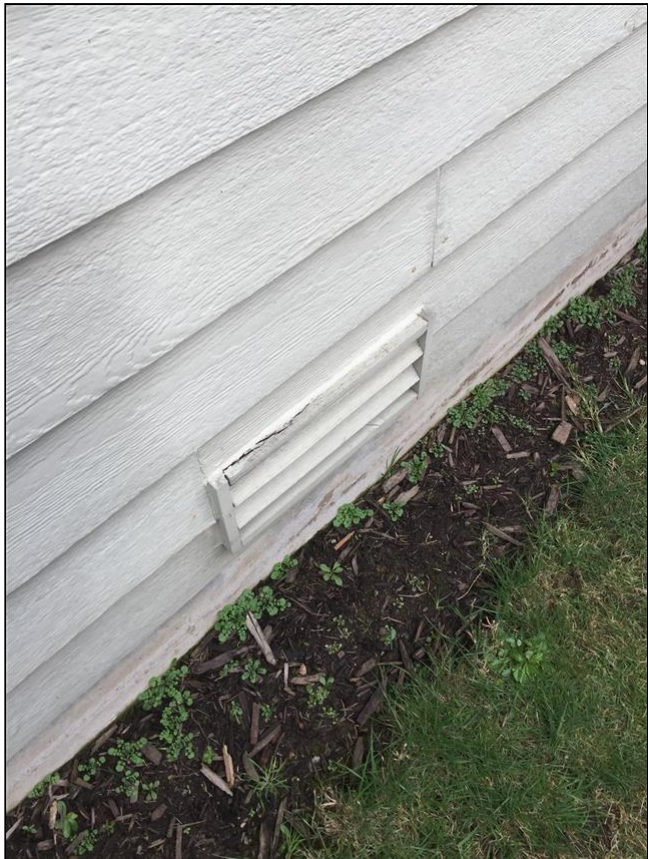
1.0 Item 9(Picture) Vent trim board damage
