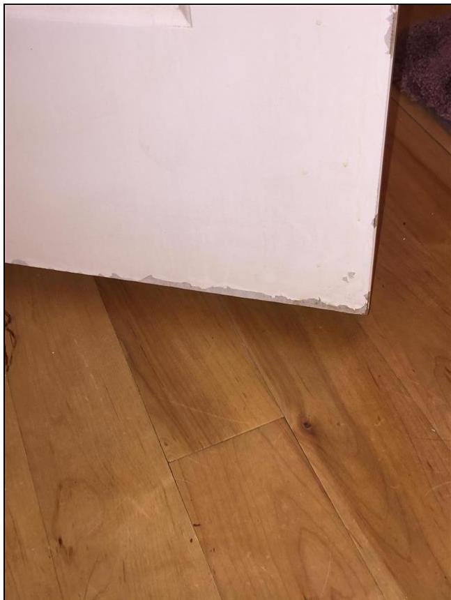
4.3 Item 1(Picture) Bottom of bathroom door damage
